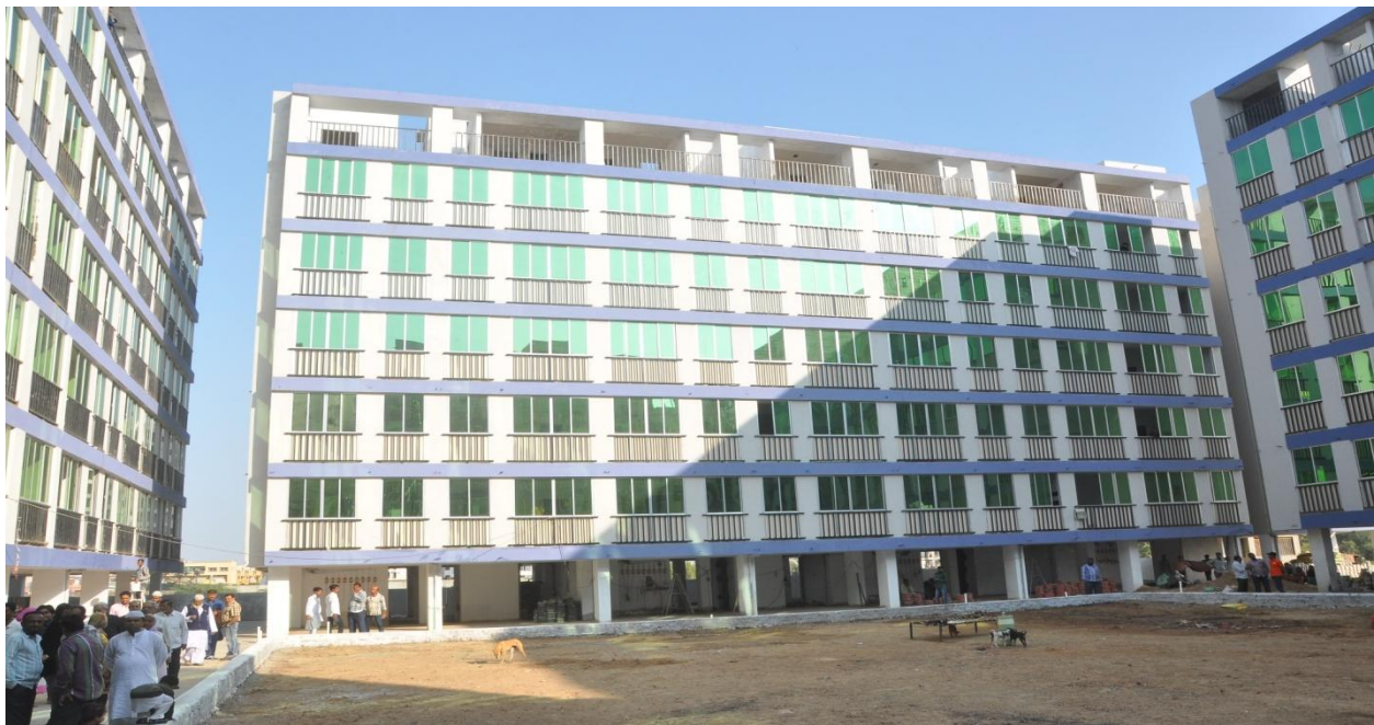
Taybah Residence, Ahmedabad: 60 apartments booked for our stake holders.
